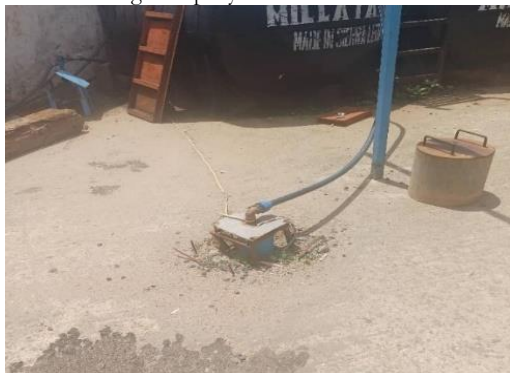
Figure 7: Unprotected & Unmetered Water Inlet Point at M.R Distilleries
