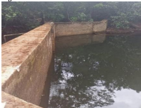
Figure 8: Casted and Unmetered Water Inlet Point at Rainbow Paints.
