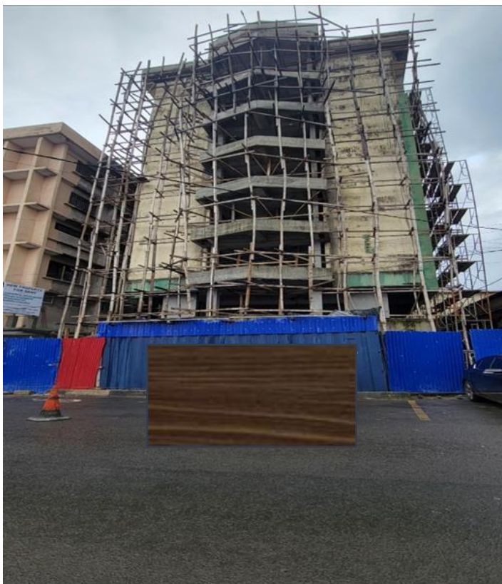
Unfinished structure of Marong House - Charlotte Street
