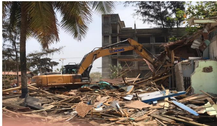
Photo of demolition exercise at the beach
