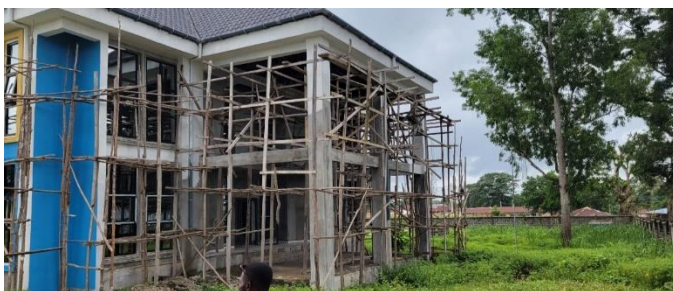
Unfinished Structure of the Moyamba District Office
