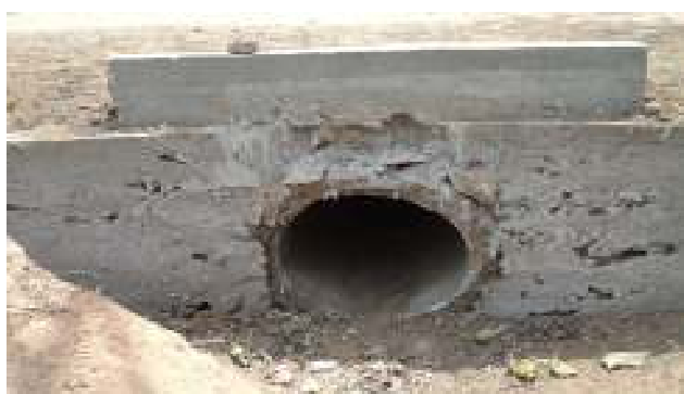
Poorly plastered pipe culvert (pic. 17)
