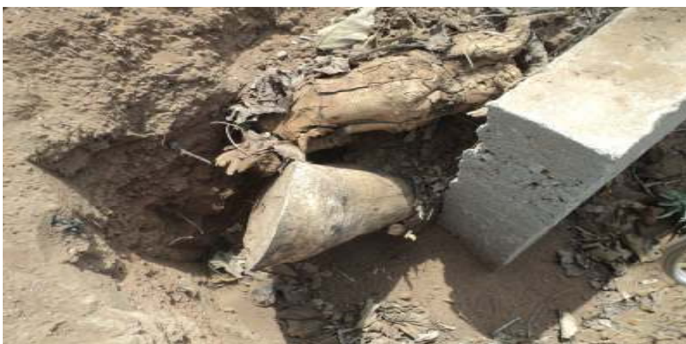
Logs used to backfill a culvert at Makump to Kangbatama, Port Loko District (pic. 12)
