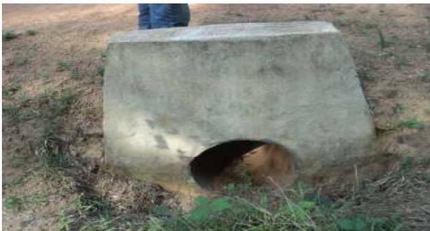
A pipe culvert without wing walls at Port Loko – Gberay Bana Road
