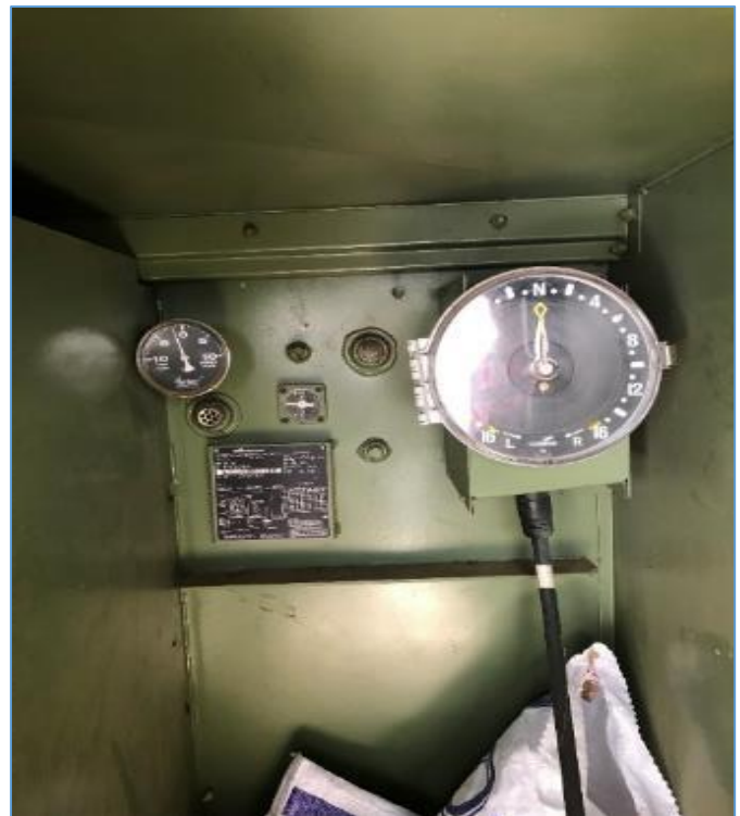
Picture 24: Inoperable 165KVA voltage regulator
