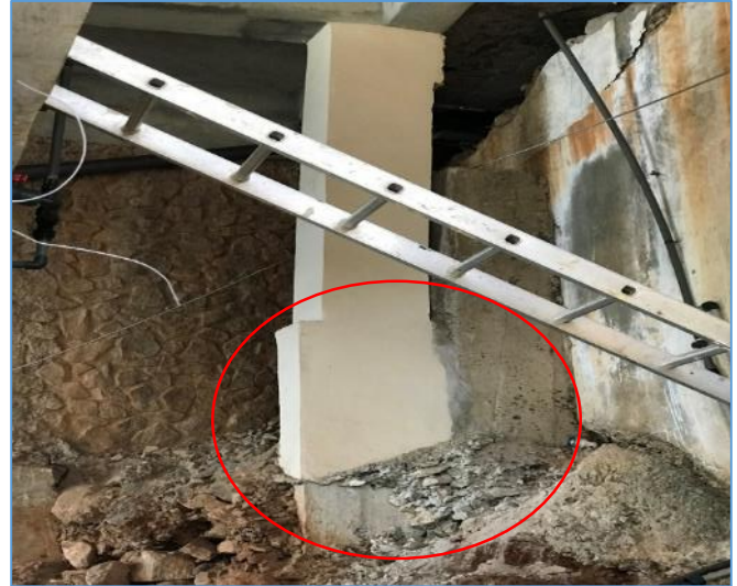
Picture 28: Poorly supported retaining wall footing and column
