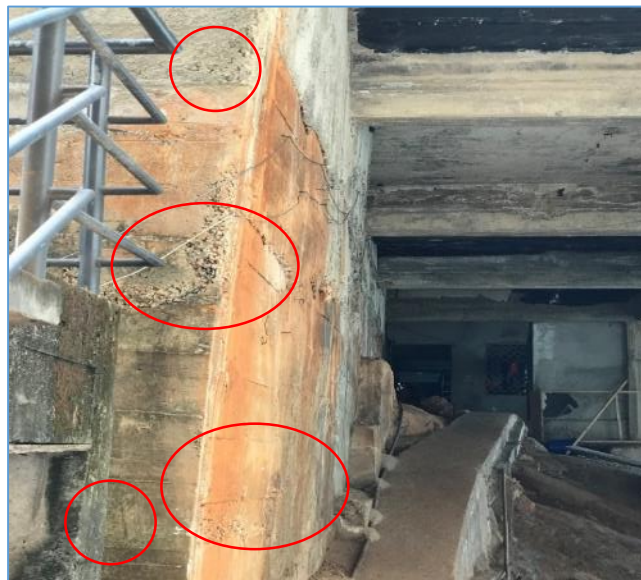
Picture 34: Honeycombing in columns
