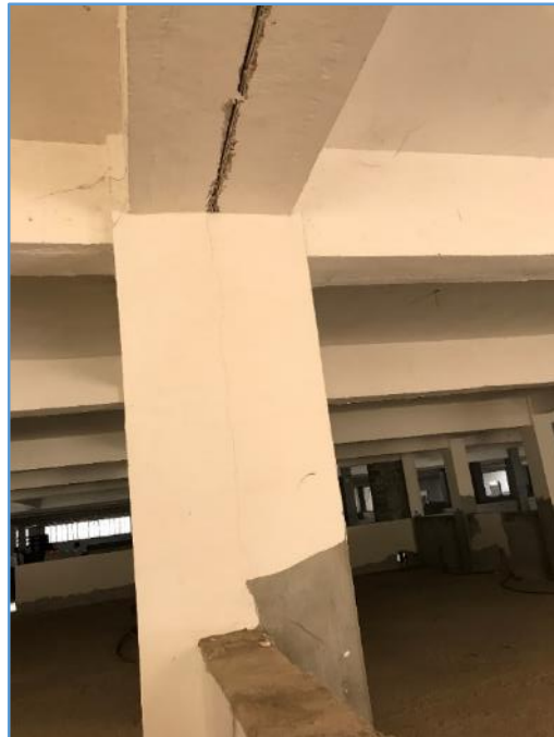
Picture 126: Expansion joint in beams
