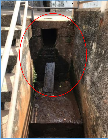
Picture 27: Poorly supported retaining wall footing and column
