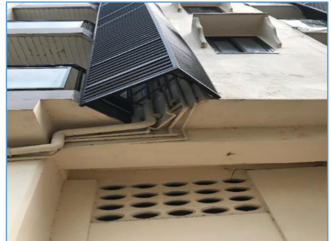
Picture 18: Poor connection of external pipelines
