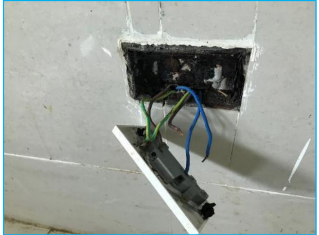
Picture 100: poorly installed wall socket with corroded pattress box
