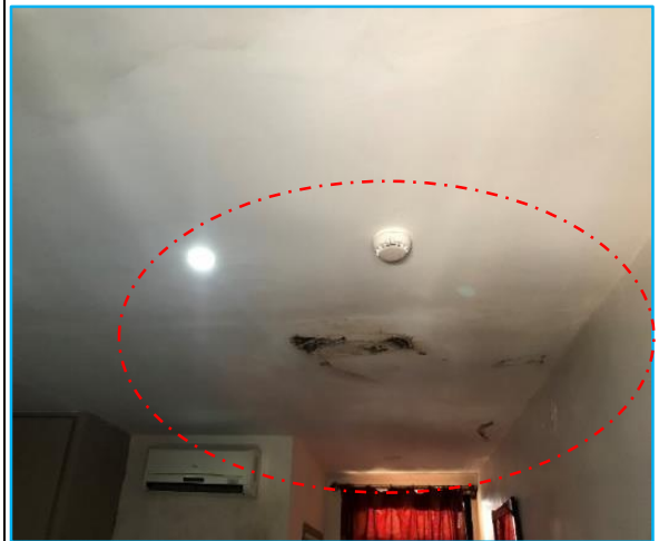
Picture 10: Crack in ceiling of hotel room
