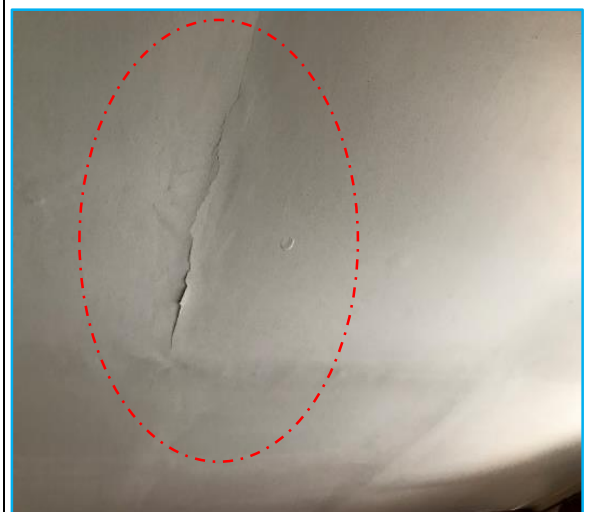
Picture 10: Crack in ceiling of hotel room
