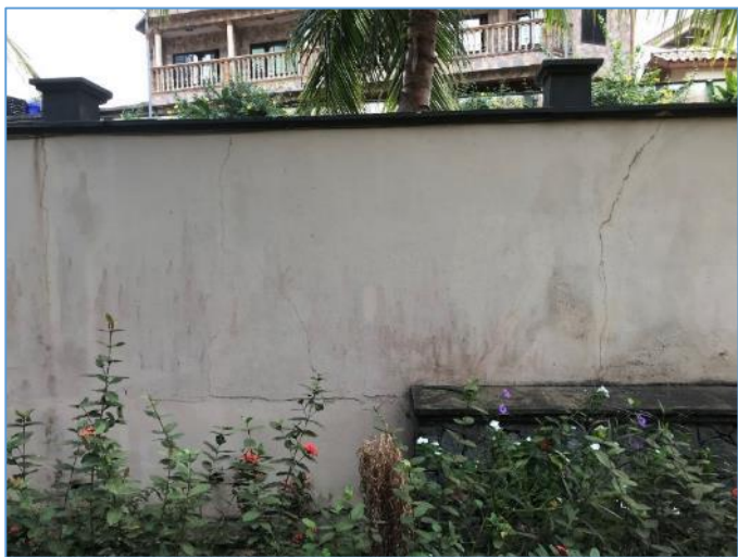
Picture 41: Cracks in external fence wall
