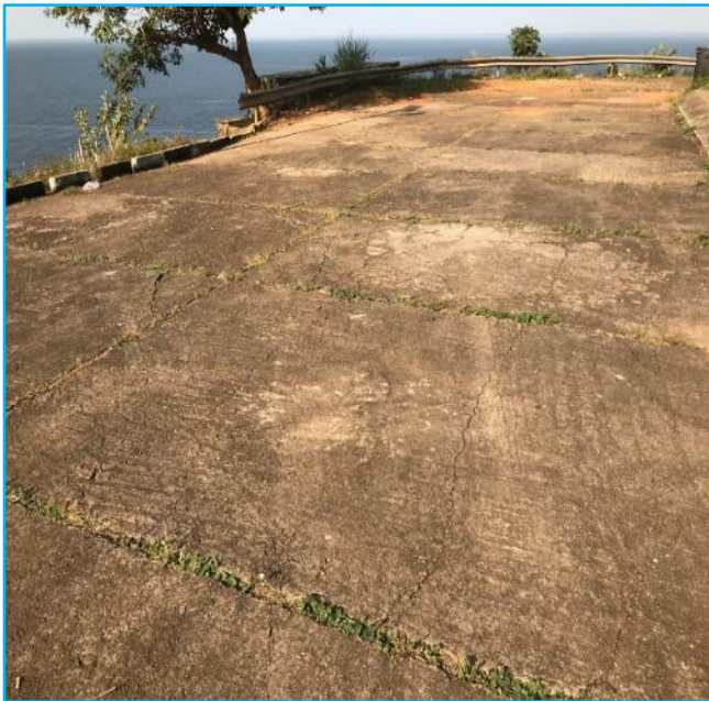
Picture 101: Cracks in concrete drive way behind conference centre
