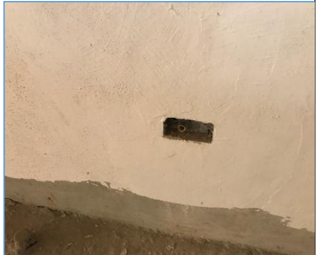
Picture 116: Electrical works not completed (pattress boxes and PVC pipes installed without electrical wiring and fixtures)
