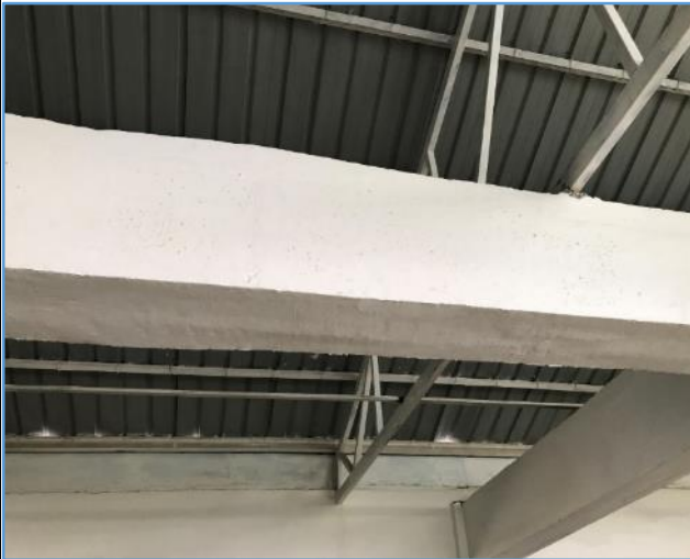
Picture 123: Beams constructed are rendered but not horizontally plumbed.
