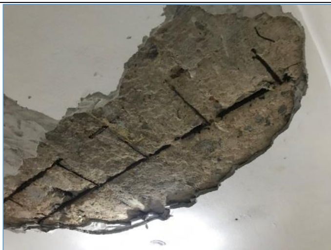
Picture 40: Failed concrete cover exposing rusted reinforcement in slabs
