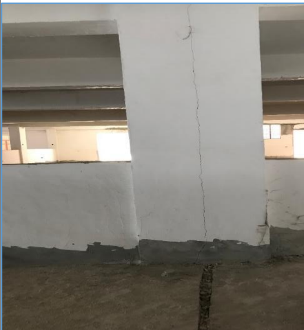
Picture 127: Expansion joint in column sealed with
