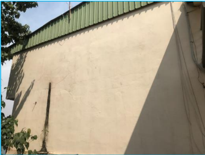
Picture 7: Cracks and dampness in external walls
