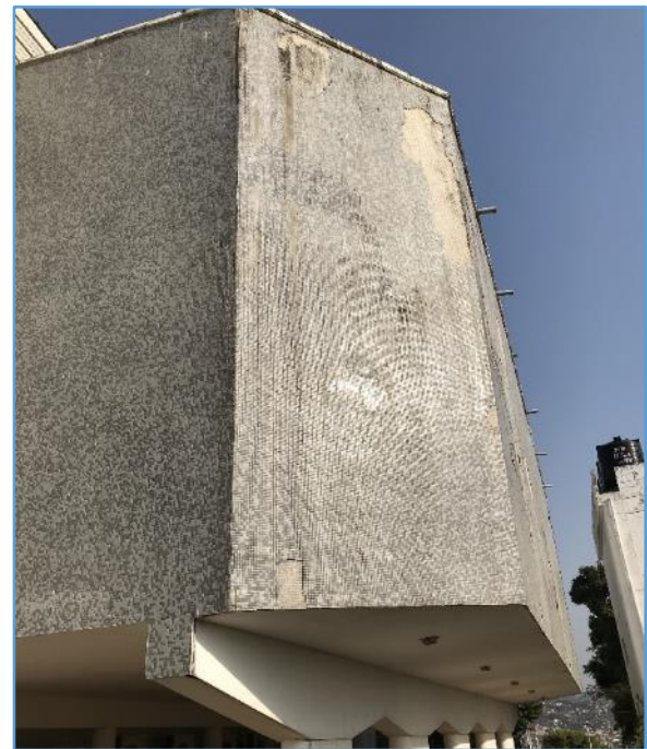
Picture 102: loose external wall tiles fallen off
