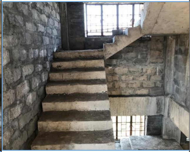
Picture 150: Honey combing observed in staircase
