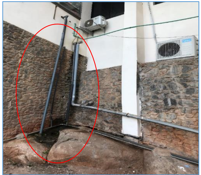
Picture 16: Poor connection of sewage pipelines
