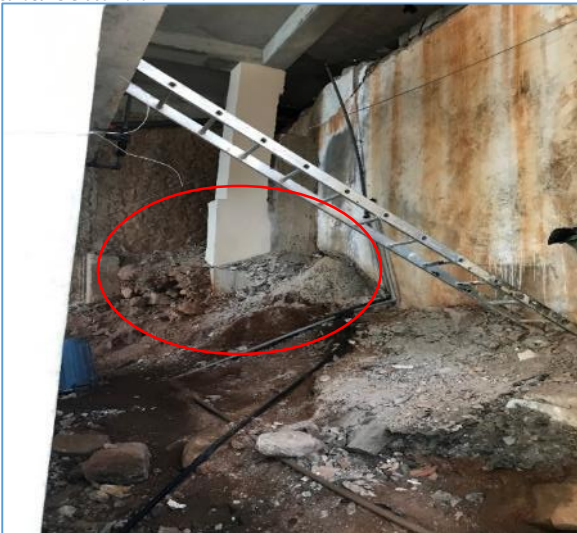
Picture 27: Poorly supported retaining wall footing and column
