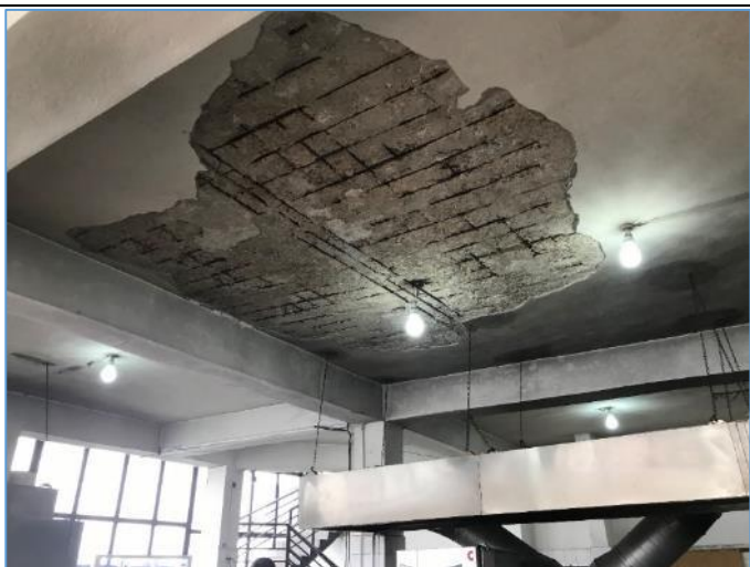
Picture 39: Failed concrete cover exposing rusted reinforcement in slabs
