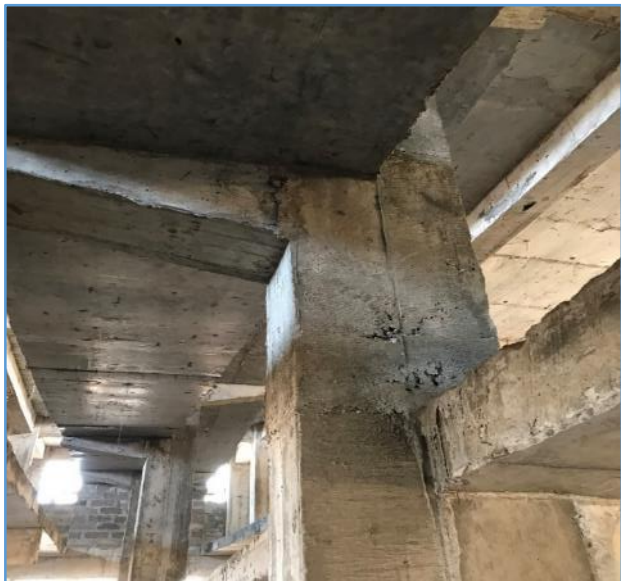
Picture 145: Honeycombing seen in reinforced concrete columns, beams, slabs and staircase
