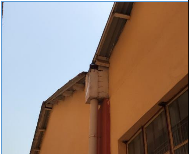
Picture 120: Rain water roof drain fitted with steel collector (instead of plastic) and fitted to PVC pipe
