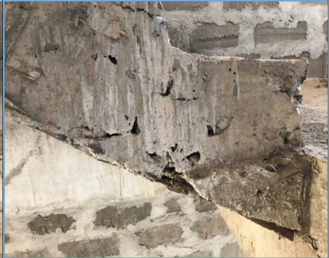
Picture 150: Honey combing observed in staircase
