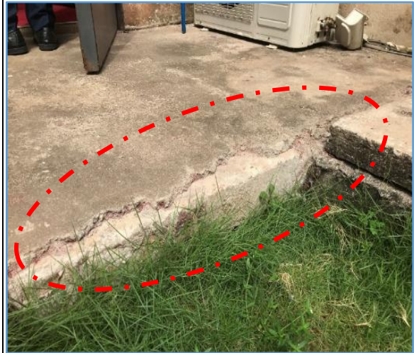
Picture 12: Deteriorated mortar screed on floor leading to garden view
