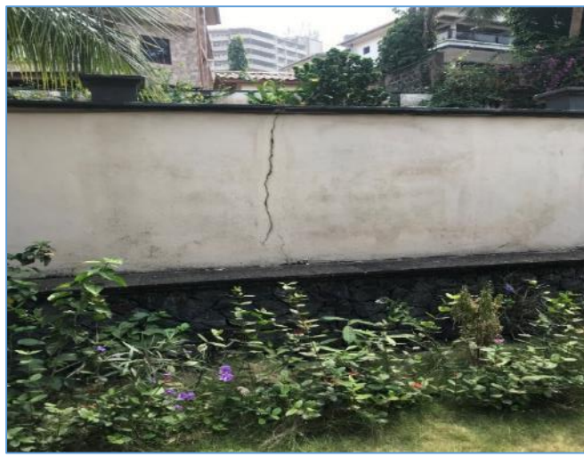
Picture 42: Cracks in external fence wall
