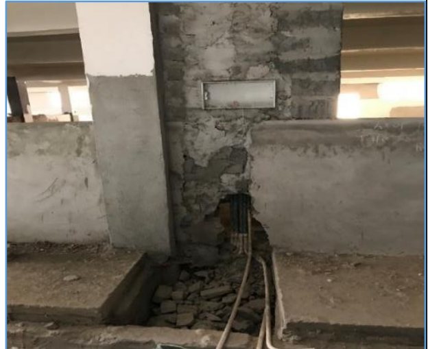
Picture 118: Electrical works not completed (pattress boxes and PVC pipes installed without
