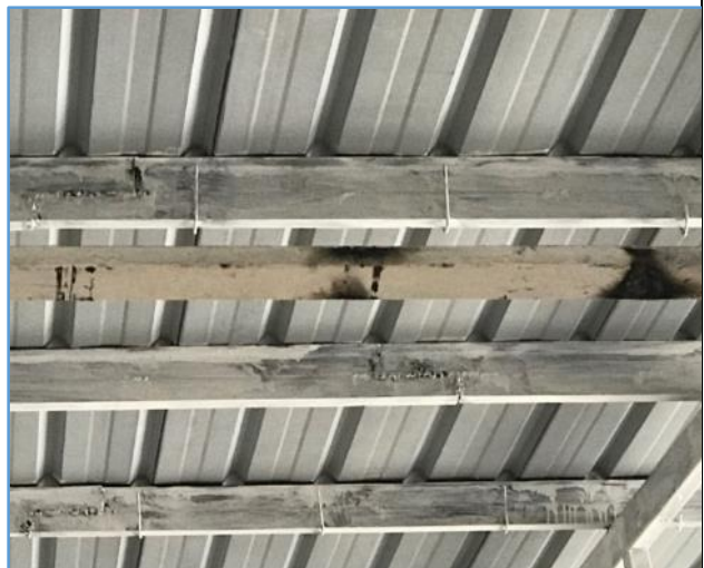
Picture 134: Welded Steel truss and roof hooks not does not conform to drawings provided
