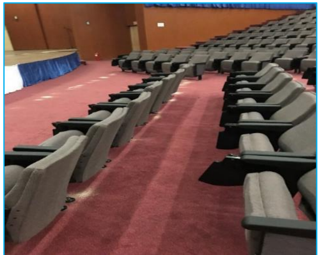
Picture 86: Wood boring insect residue left on carpet in main auditorium
