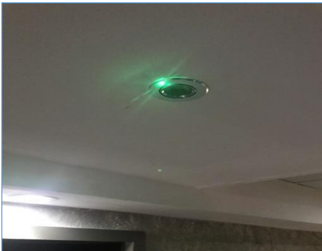
Picture 69: Emergency lights installed
