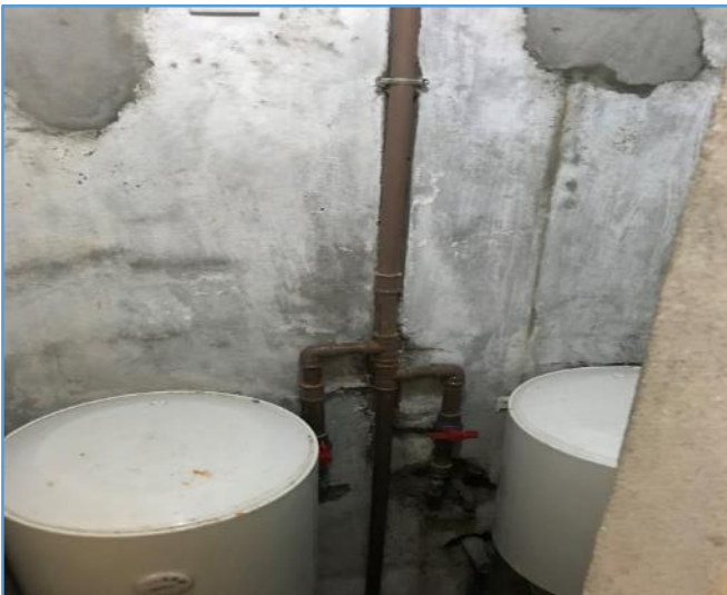
Picture 13: Poor connection of hot water pipelines
