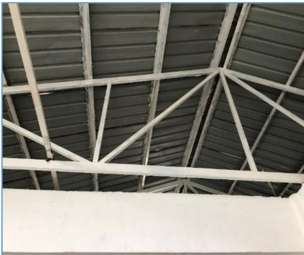
Picture 133: Lapping of roofing sheet not done right leaving hole for rain water to enter the building
