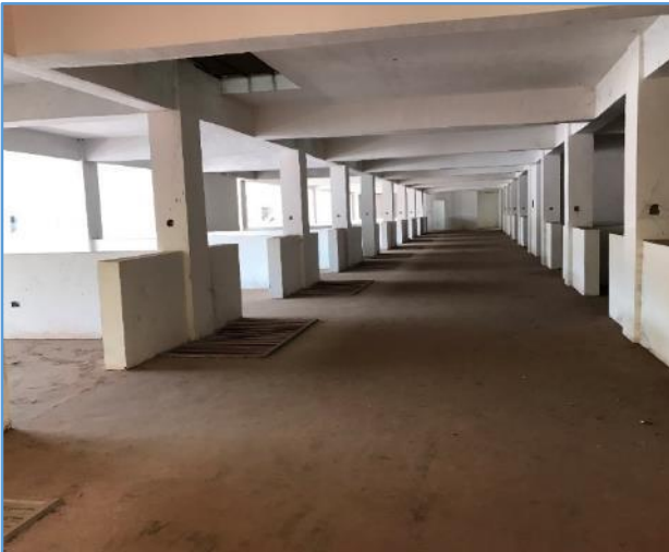
Picture 115: Electrical works not completed (pattress boxes and PVC pipes installed without electrical wiring and fixtures)
