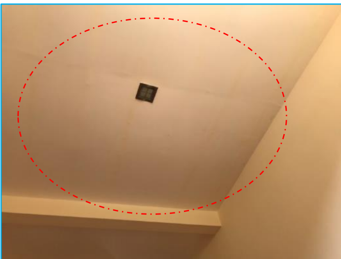
Picture 9: Signs of water leakage in hotel room ceiling
