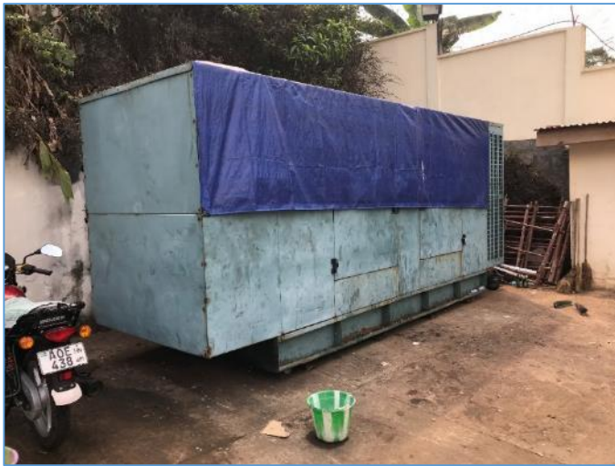
Picture 23: Inoperable 165KVA voltage regulator
