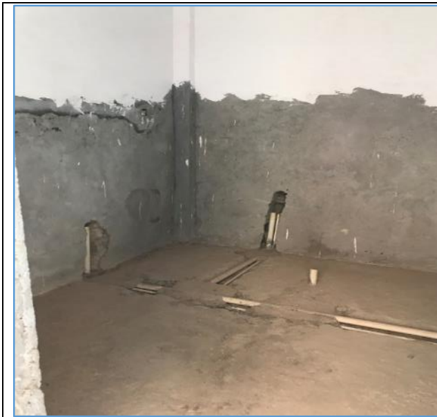
Picture 115: Electrical works not completed (pattress boxes and PVC pipes installed without electrical wiring and fixtures)
