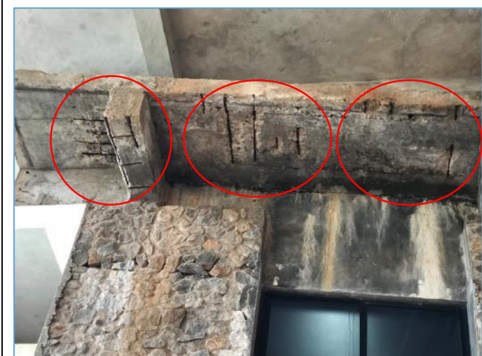
Picture 35: External beam and slab with rusted reinforcement exposed
