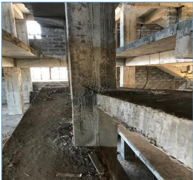
Picture 146: Honeycombing seen in reinforced concrete columns, beams, slabs and staircase
