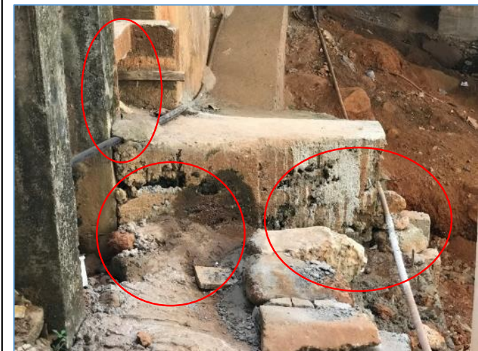
Picture 31: Honeycombing in concrete works
