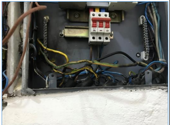
Picture 20: Unprofessional wiring of electrical mains switch
