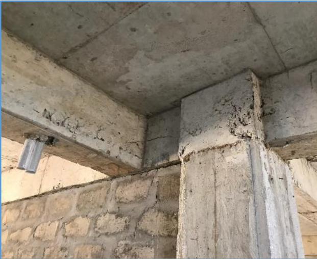
Picture 149: Honeycombing observed in column and beam
