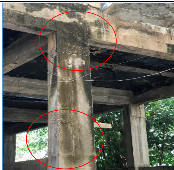
Picture 36: Dampness in beams at Gym
