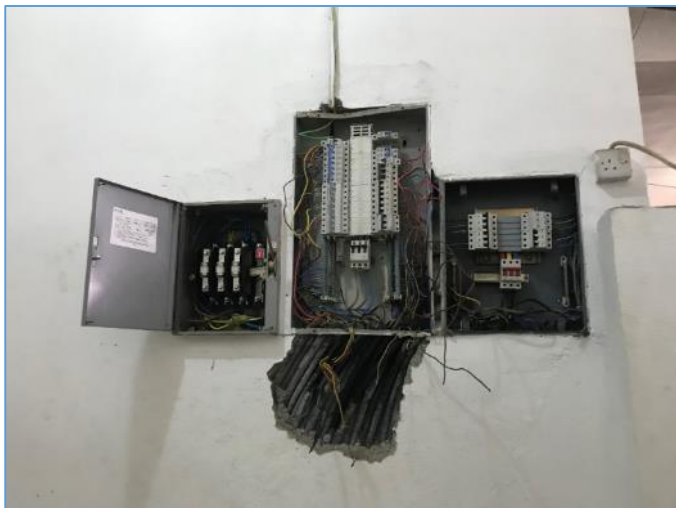
Picture 19: Unprofessional wiring of electrical mains switch
