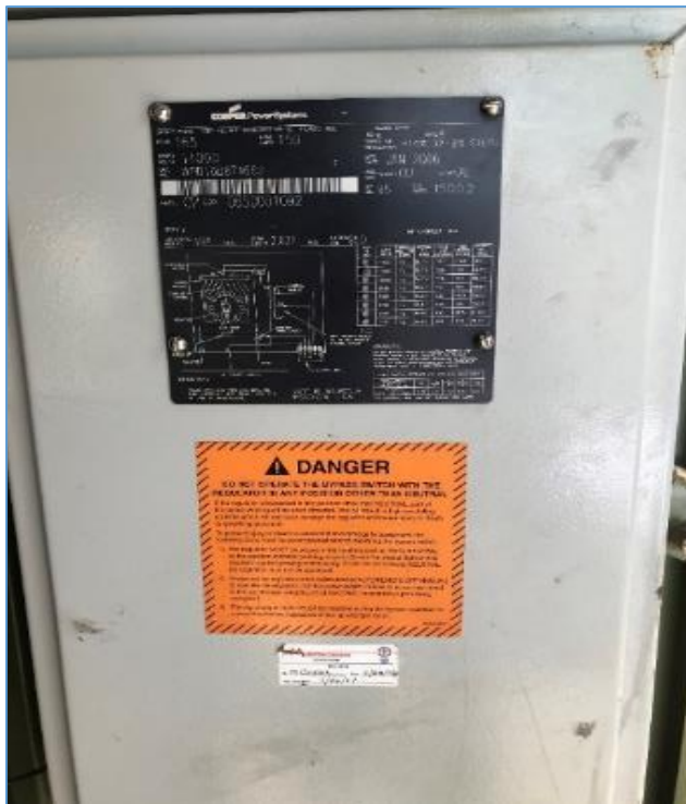
Picture 23: Inoperable 165KVA voltage regulator
