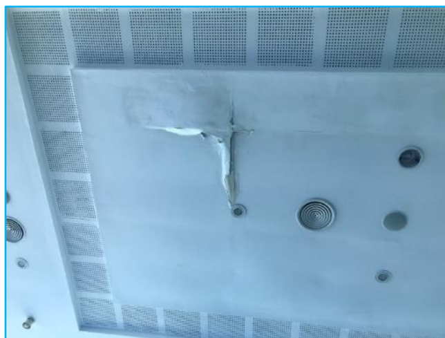
Picture 82: Damaged ceiling at Banquet Hall
