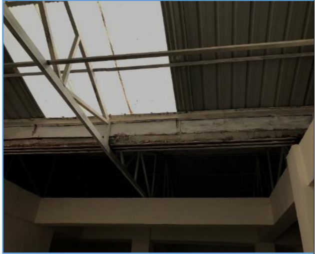
Picture 138: Fabricated steel rain gutter in between
