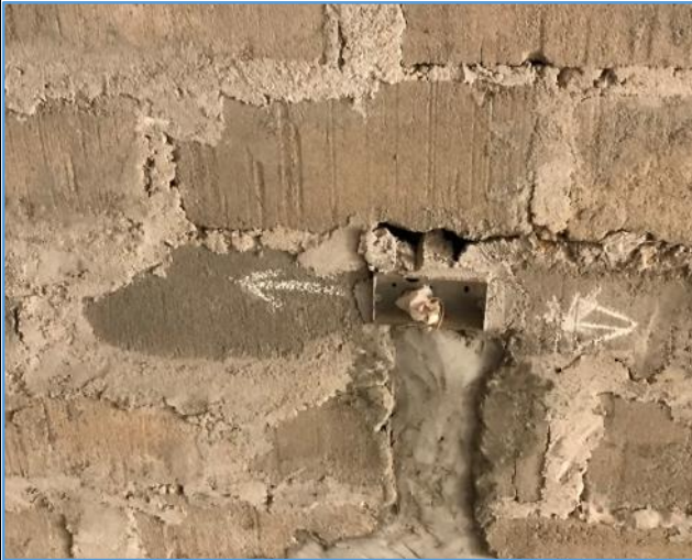
Picture 117: Electrical works not completed (pattress boxes and PVC pipes installed without
