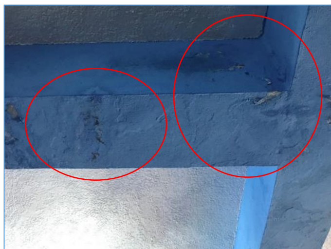
Picture 36: Dampness in beams at Gym
