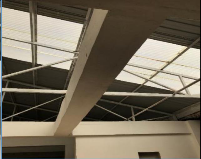
Picture 124: Horizontally unplumbed beams
