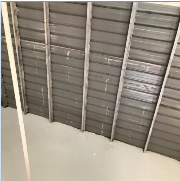
Picture 137: Poorly fitted long span roof with hole
