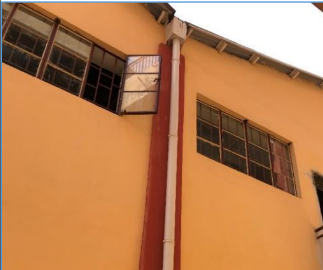
Picture 119: Rain water roof drain fitted with steel collector (instead of plastic) and fitted to PVC pipe
