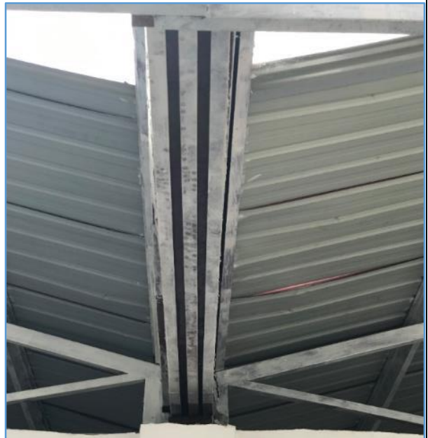
Picture 138: Fabricated steel rain gutter in between
