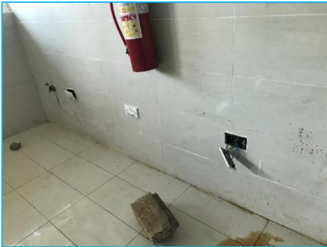
Picture 99: Poorly installed electrical fittings in Kitchen 2
