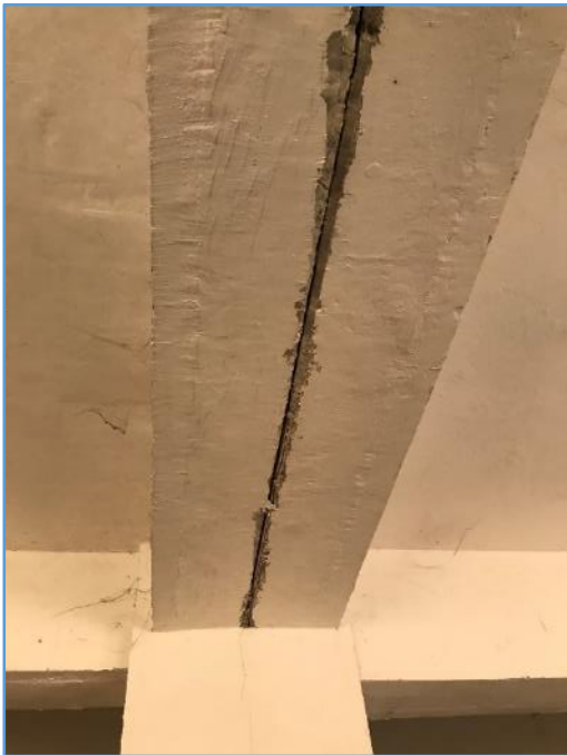
Picture 125: Expansion joint in beams
