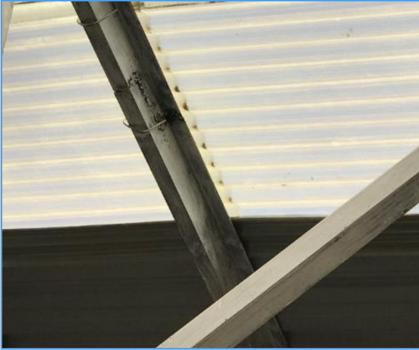
Picture 137: Poorly fitted long span roof with hole
