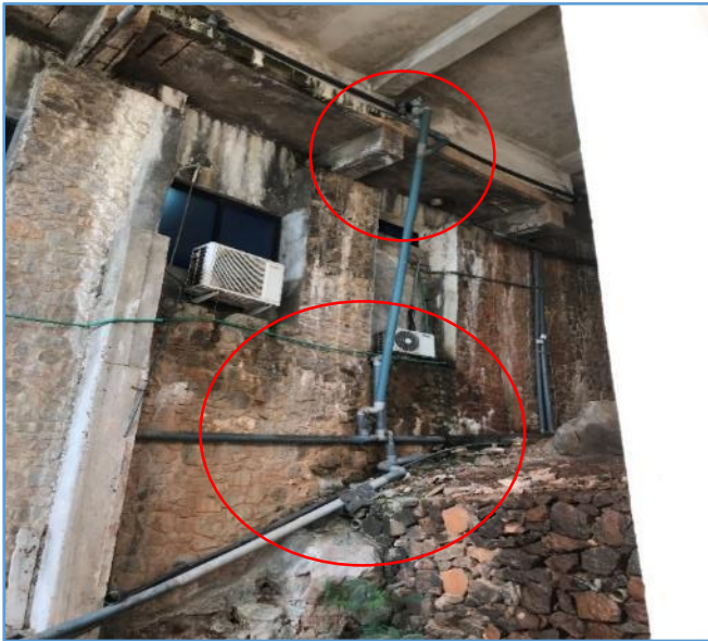
Picture 17: Poor connection of internal pipelines
