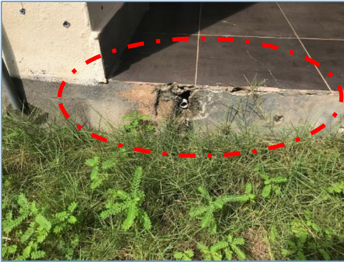
Picture 11: Deteriorating floor tiles
