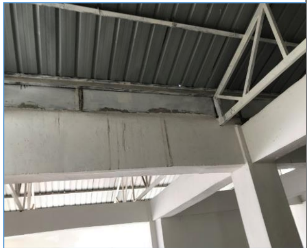
Picture 134: Welded Steel truss and roof hooks not does not conform to drawings provided
