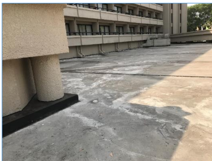
Picture 54: Resealed of concrete roof on top of conference and meeting rooms
