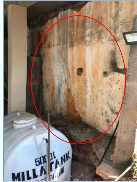
Picture 26: Cracks in retaining wall
