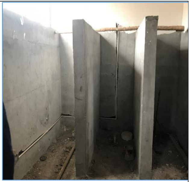
Picture 116: Electrical works not completed (pattress boxes and PVC pipes installed without electrical wiring and fixtures)
