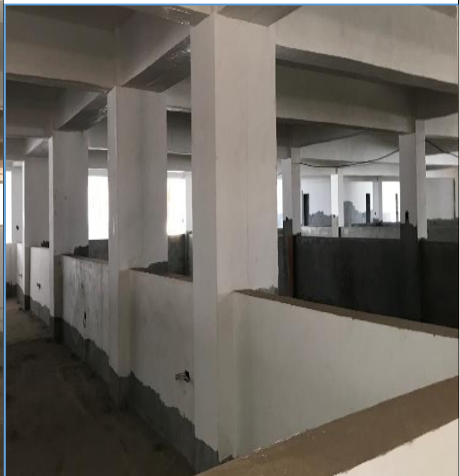
Picture 128: Columns with expansion joints covered with mortar showing cracks
