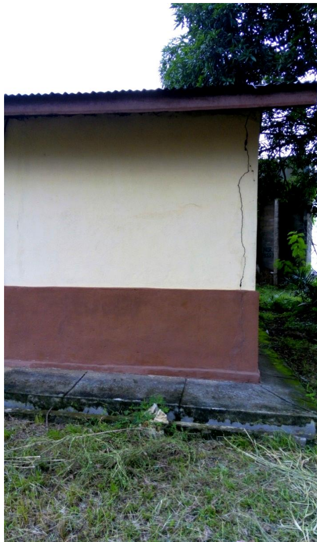
Photo of a crack in the wall of a MAFFS store. The cracks expose the Fertilizer to the elements . Photo taken on 22 nd June, 2017.
