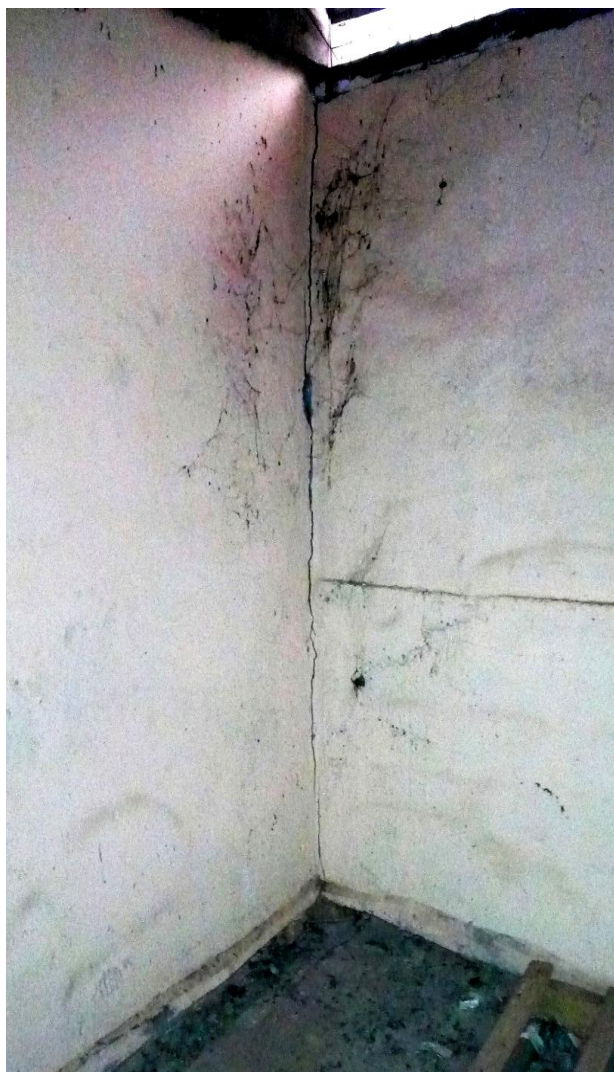
Photo of the cracks in the wall of one of MAFFS' stores . The cracks expose the Fertilizer to the elements. Photo taken on 22 nd June, 2017.
