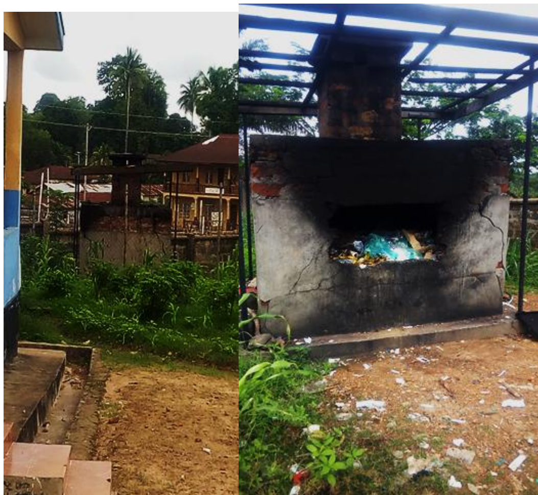
Photo: locally constructed incinerator within the Bo government hospital, and very close to residential area; 9 th June 2017
