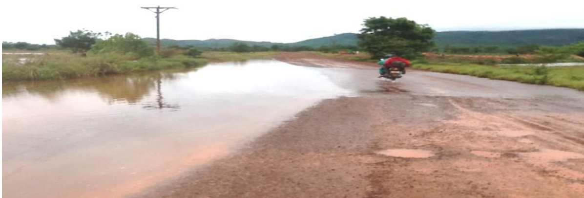
Photo No. 2. Flooding on the road between two mined out pits in Moyamba district – photo taken in June, 2015
