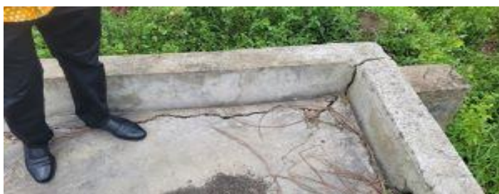
Cracks in constructed dry floor at Gandorbun village, Niawa Chiefdom, Kenema District
